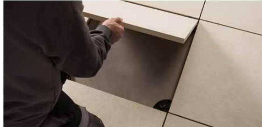
**LOW HEIGHT SUPPORTS (UP TO 3/4" - 20 MM) PEDESTAL INSTALLATION OVER EXISTING SUBSTRATE**
