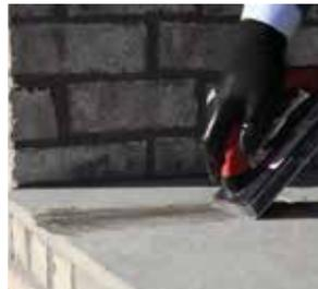
PIC 1. Fill joint with grout.
