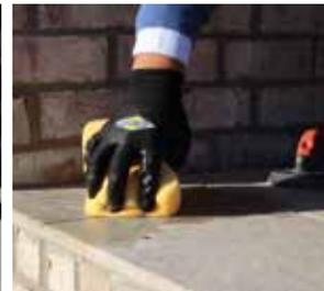
PIC 2. Remove excess grout with clean water.
