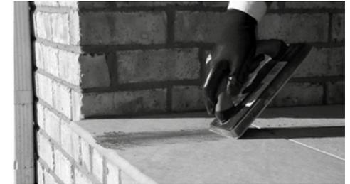
PIC 2. Remove excess grout with clean water.
