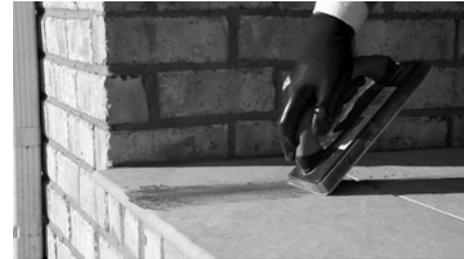
PIC 1. Fill joint with grout.
